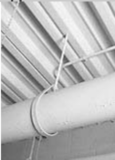
Hanging threaded rods for pipe suspension
