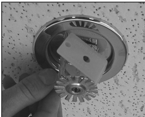
Figure 1: Sprinkler shield being removed from a pendent sprinkler.
